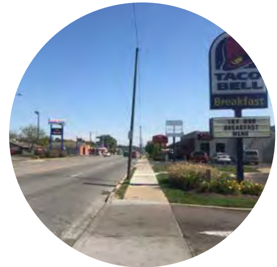
Nondescript commercial corridors with a deteriorated public realm present one of the County's greatest opportunities for enhanced character.
