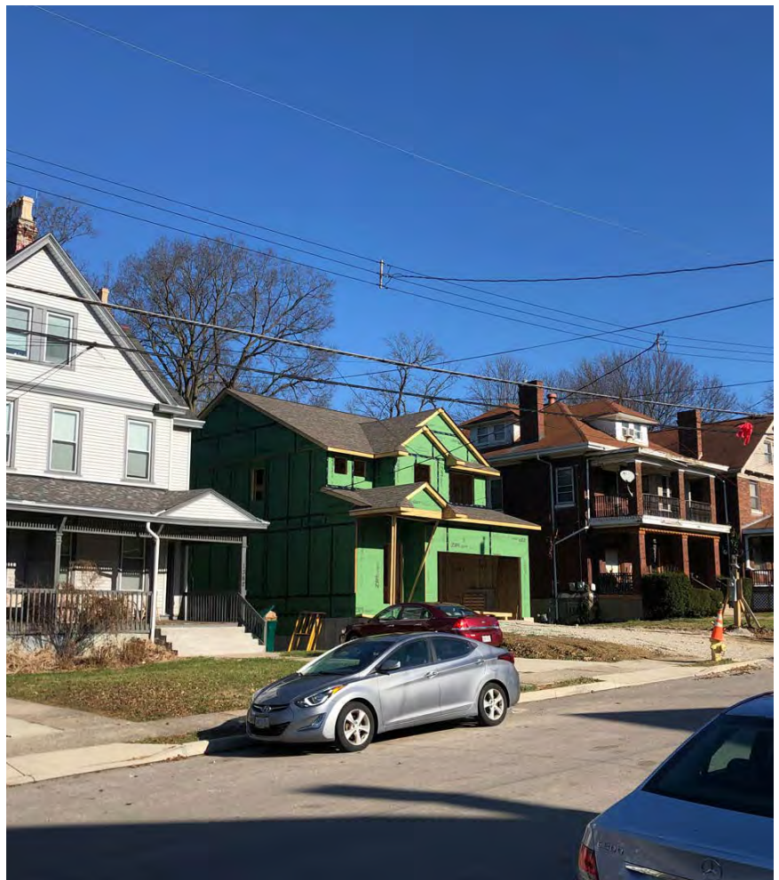
Progress is often best shown with new construction.
