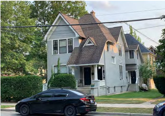
An example of a three-unit building that fits into a single family neighborhood
