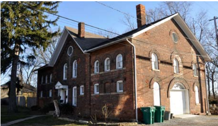
[ PHOTO 2 ] A large brick carriage house on East High Street.
