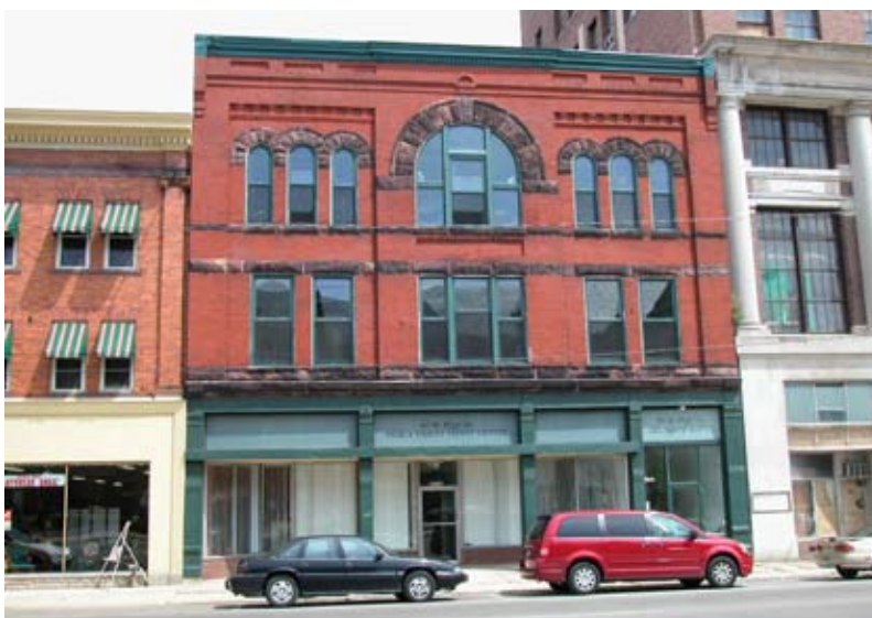
[ PHOTO 2 ] This High Street building is an example of an upper facade topped by a simple parapet with very shallow projection. The sandstone trim and arched wood windows are significant character-defining features of the building.
