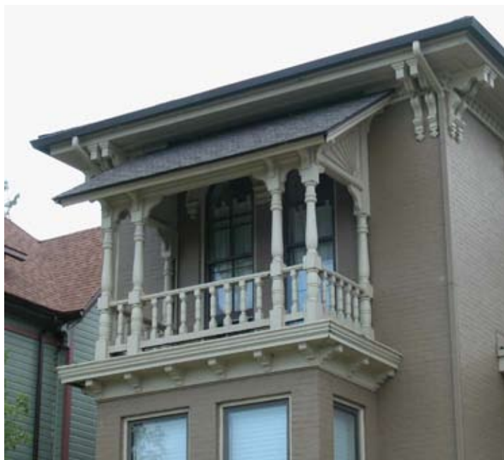
[ PHOTO 4 ] A distinctive second story porch.
