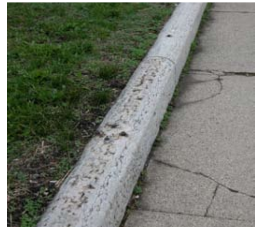
[ PHOTO 9 ] Original limestone curbing on East High Street.
