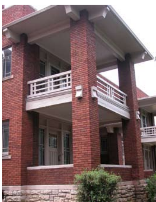
[ PHOTO 5 ] Two-story brick porch on Craftsman style apartment building.
