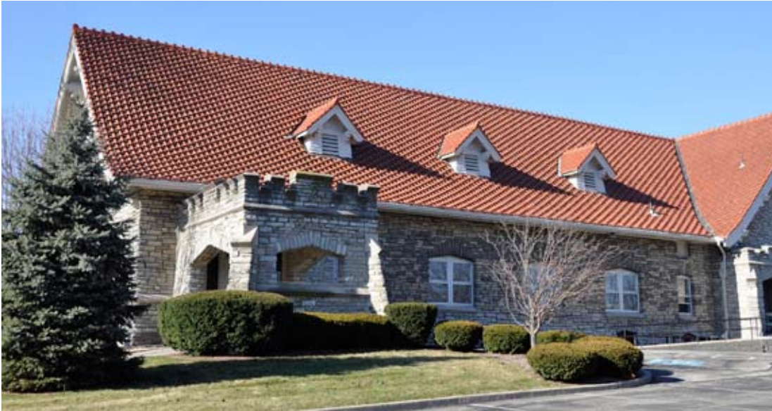
[ PHOTO 3 ] A distinctive example of a clay tile roof in Springfield
