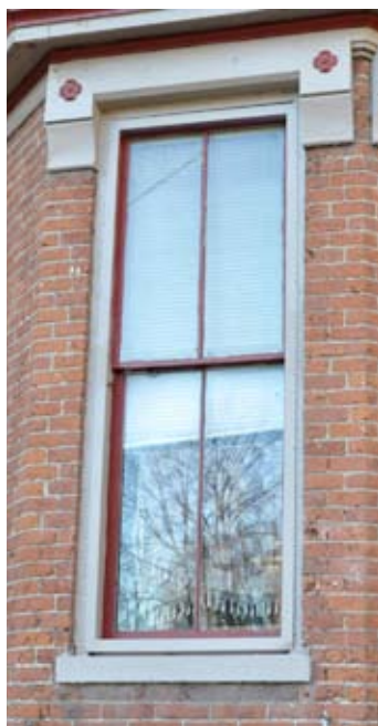
[ PHOTO 2 ] A historic 2-over-2 pane window.
