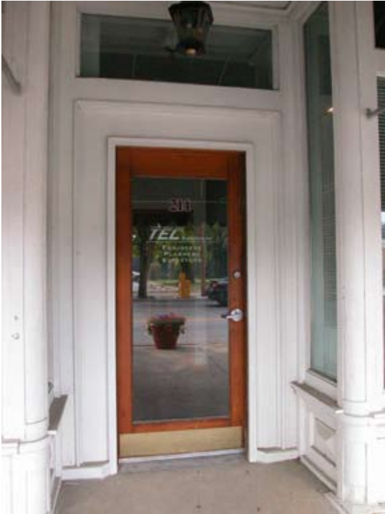
[ PHOTO 7 ] Commercial doorway.
