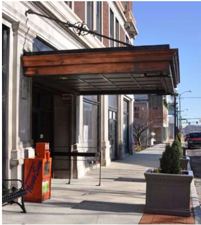
[ PHOTO 4 ] An example of a traditional projecting fixed canopy on a downtown commercial building.
