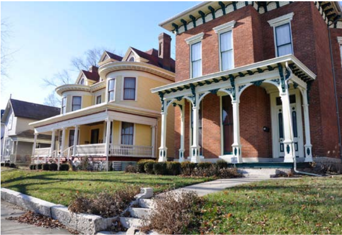
[ PHOTO 1 ] Porches along South Fountain Avenue.
