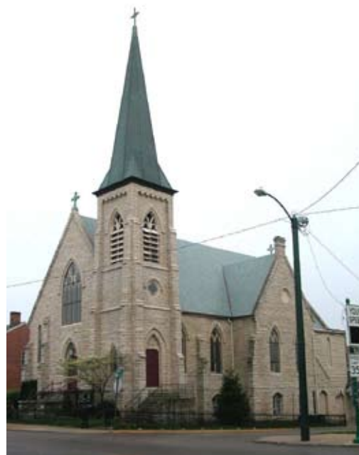
[ PHOTO 28 ] 403 E. High Street (Late Gothic Revival)
