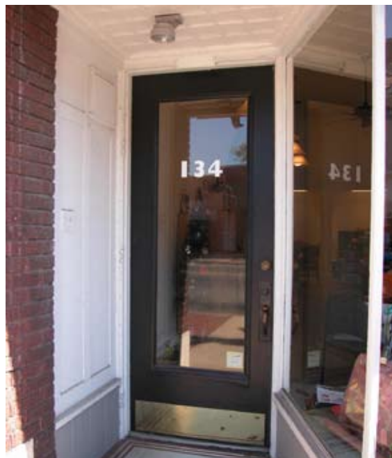
[ PHOTO 12 ] A full light commercial door is usually the best choice for a historic storefront.
