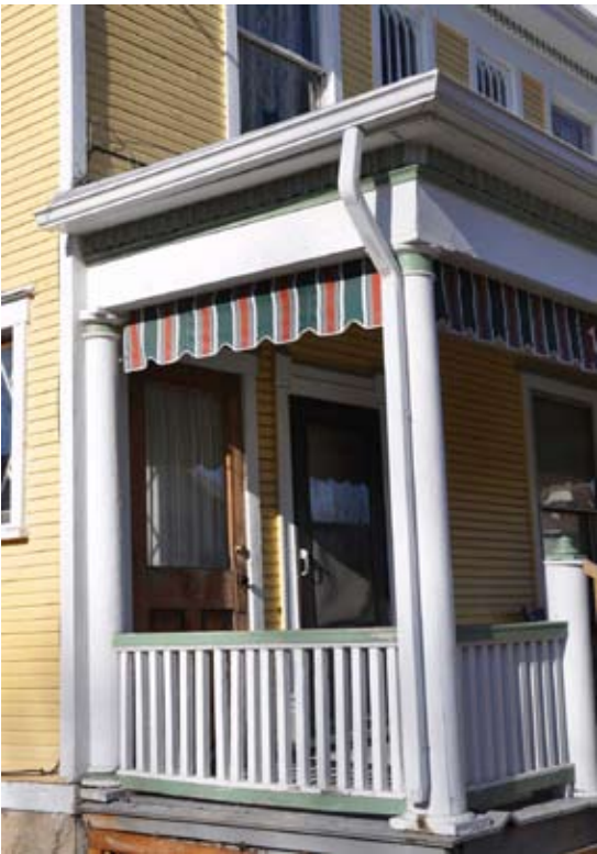
[ PHOTO 3 ]: Although not as common as storefront awnings, residential awnings at a porch may be appropriate when kept extremely simple and restrained.
