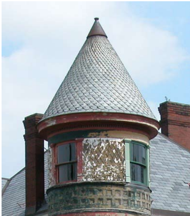
[ PHOTO 8 ] A historic conical roof is a significant feature.
