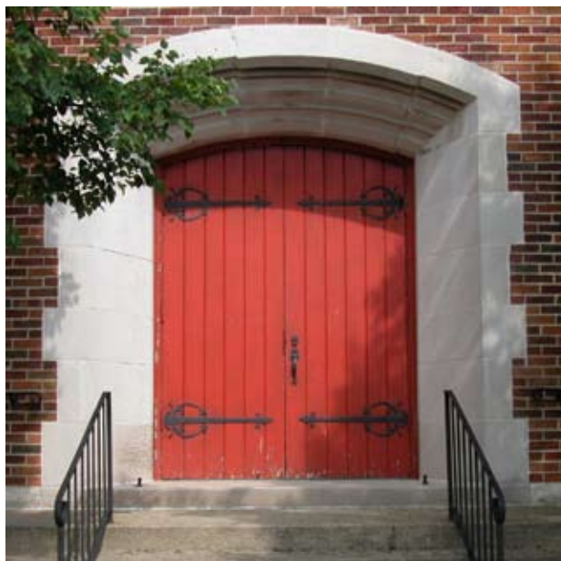
[ PHOTO 9 ] A church entrance on South Fountain Avenue.
