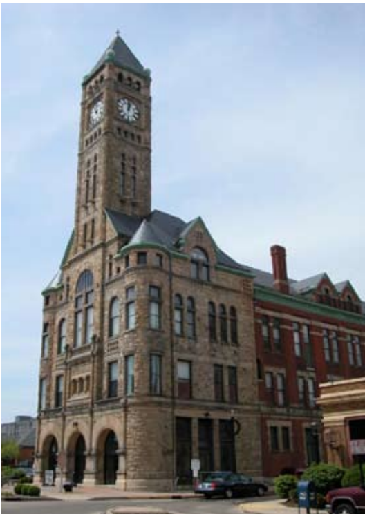
{ PHOTO 4 } Rock-faced sandstone is the construction material for the former Springfield City Building, constructed in 1890.
