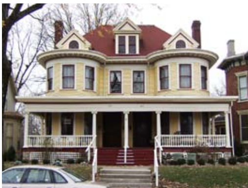
[ PHOTO 21 ] 629-631 S. Fountain (Colonial Revival double house)
