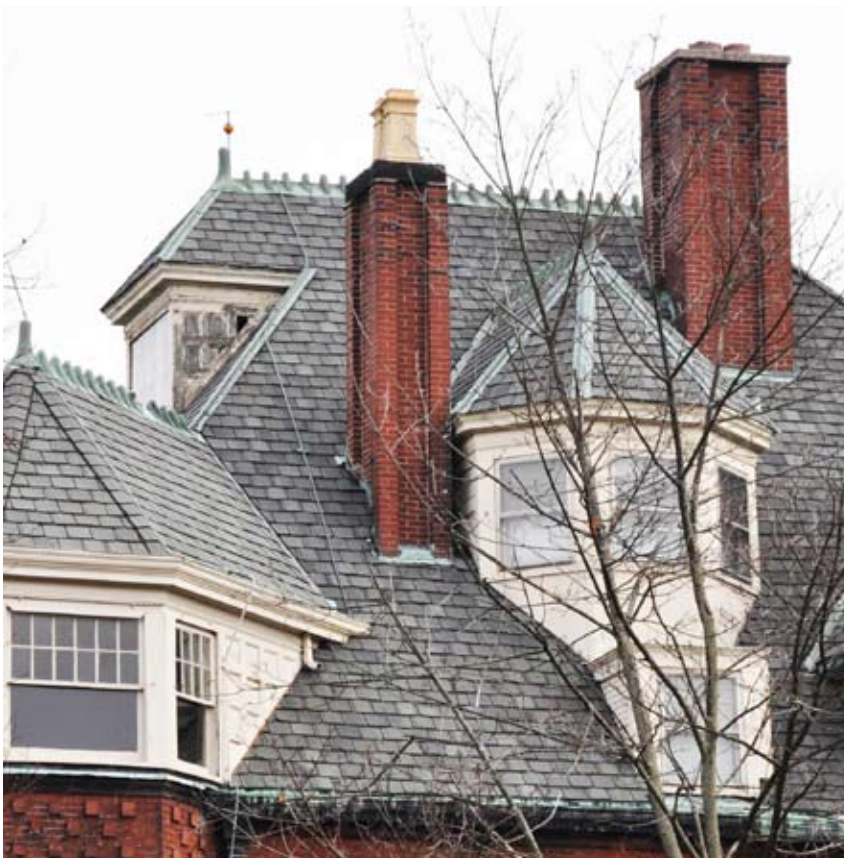
[ PHOTO 5 ] This roof replacement used a dimensional shingle that recalls the appearance of historic slate. Note how the original copper ridge caps were retained.
