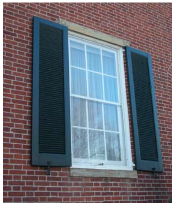
[ PHOTO 13 ] An example of historic operable window shutters.
