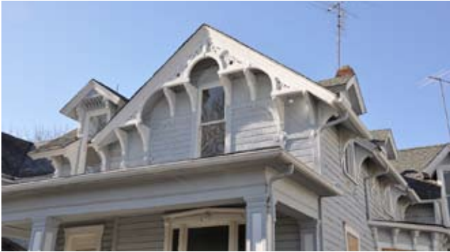
[ PHOTO 9 ] 821 S. Limestone Street (Eastlake style trim)
