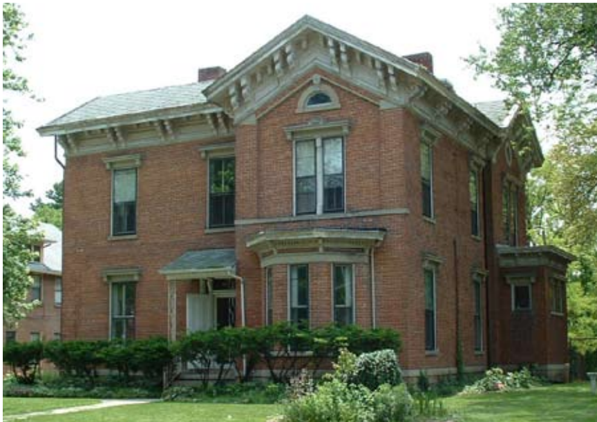
{ PHOTO 1 } A 19th century residence with brick bearing wall construction.
