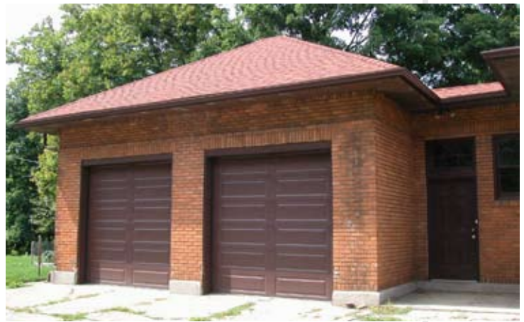
[ PHOTO 5 ] This attached 2-car garage repeats the materials and features of the main house. The connecting piece is subsidiary to both buildings. The continued use of two separate garage doors is very important.
