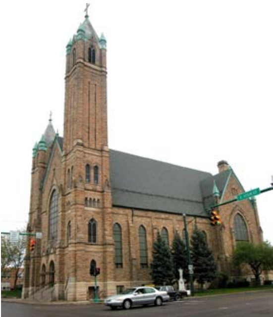
[ PHOTO 27 ] 211 E. High Street (Late Gothic Revival)
