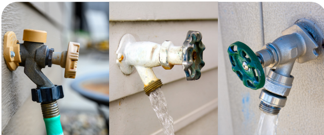
Above: Outdoor spigot with anti-siphon valve (l), hose bib without vacuum breaker (m), hose bib with vacuum breaker (r)
