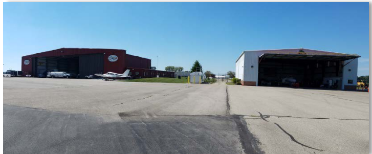
Spectra Jet Hangar #4 & Ali-Gator Air, LLC Hangar #5, Source: Woolpert, 2016. (Privately Owned Hangars)
