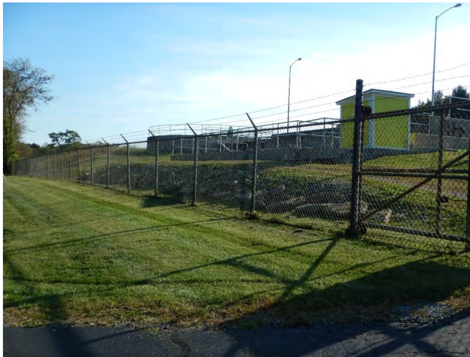
Photograph 92. Yellow Springs Waste Water Treatment Plant. Area 23 on Figure 5.
