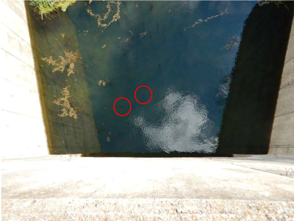
Photograph 38. Mill Creek at the inlet side of the culvert under Runway 24. Area 14 on Figure 4 showing the presence of fish within the deep water.
