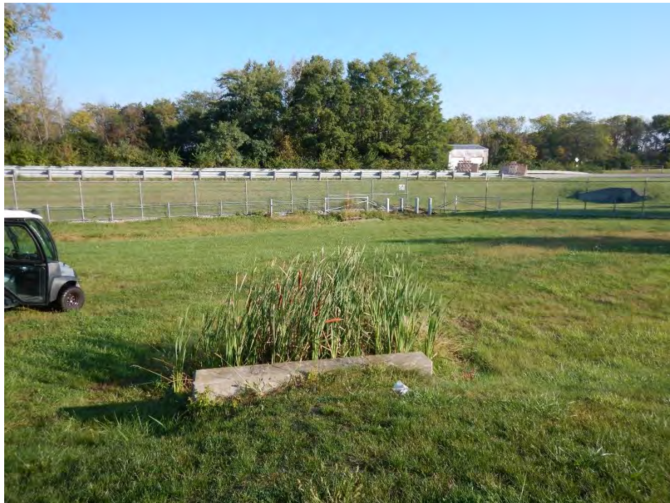
Photograph 60. Headwall and convergence of several drainages taking surface flow off the OANG base, Area 16 on Figure 4, this is near SR 794, view to the north-northeast.
