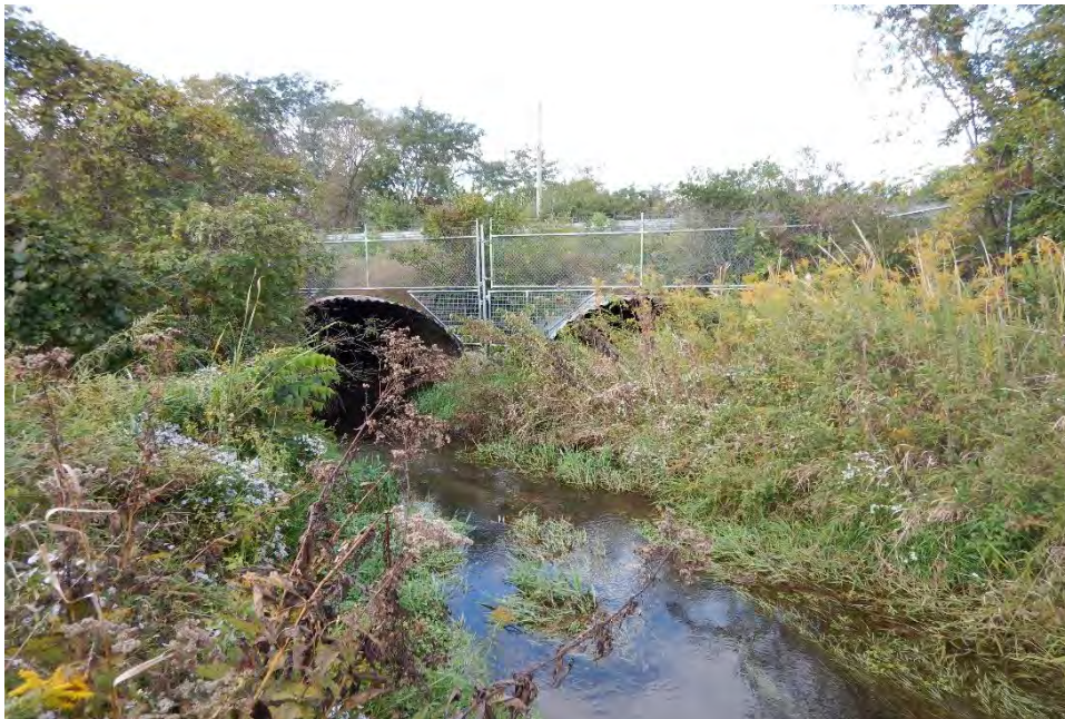
Photograph 48. Mill Creek, Area 14 on Figure 4 view to the northwest showing the culvert under Blee Road.
