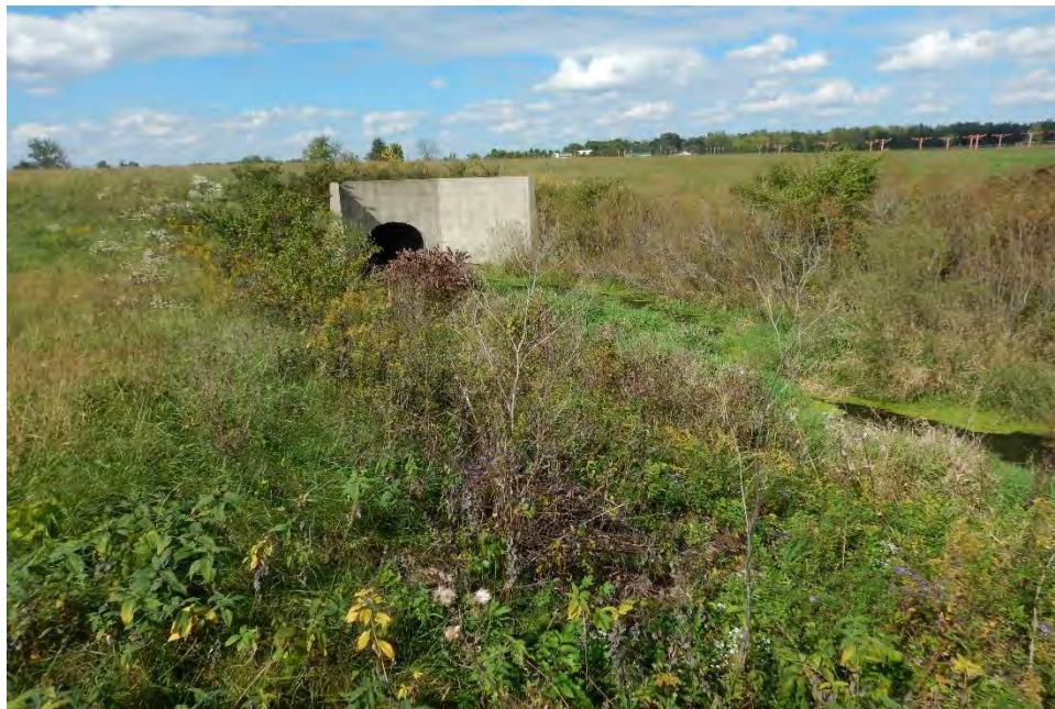
Photograph 36. Mill Creek at the inlet side of the culvert under Runway 24. Area 14 on Figure 4, view to the northwest.
