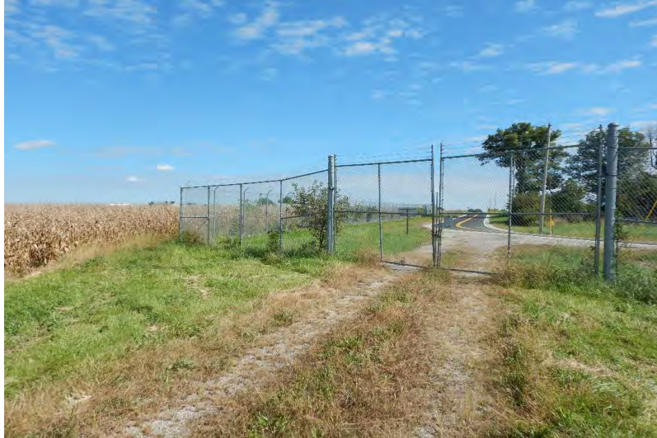
Photograph 30. The far southeast corner gate of SGH. Area 12 on Figure 4, West Jackson Road beyond the perimeter fence, view to the east.
