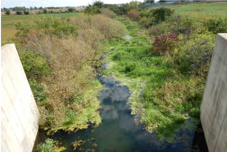
Photograph 37. Mill Creek at the inlet side of the culvert under Runway 24. Area 14 on Figure 4, view to the southeast.
