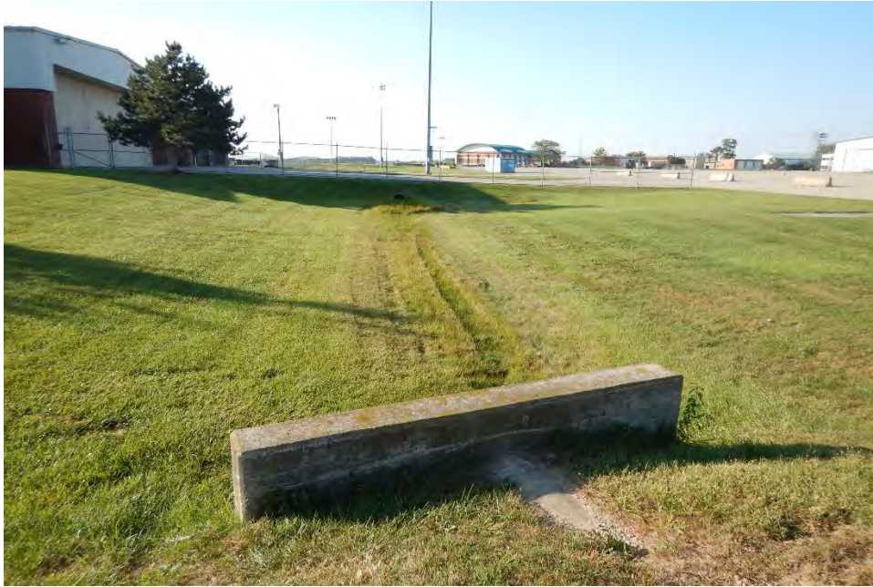
Photograph 65. Drainage swale taking surface flow off the OANG base. Area 16 on Figure 4, view to the south.
