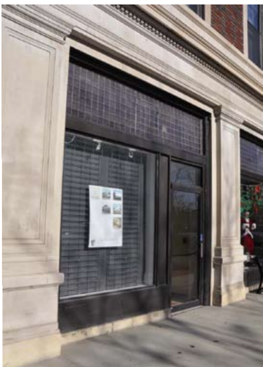
[ PHOTO 2 ] This storefront at the Shawnee Hotel retains its original prism glass transom window.
