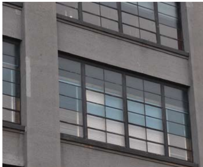
[ PHOTO 5 ] An example of an industrial style hopper window, where one section opens horizontally on a hinge for ventilation purposes.
