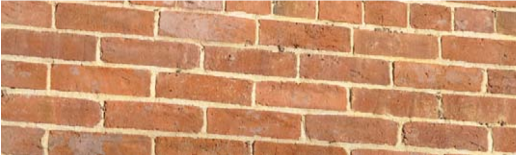
[ PHOTO 8 ] — In addition to matching the joint tooling, be sure that the mortar mix, texture and color is appropriate for the historic masonry.
