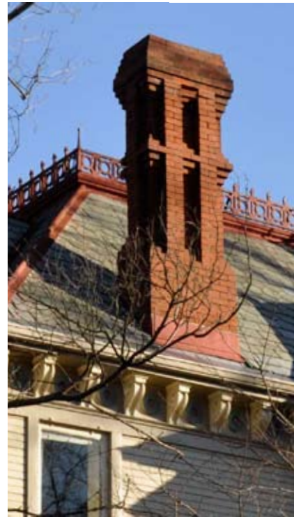
[ PHOTO 7 ] Corbelled chimney, iron cresting and ridge caps on a slate roof.
