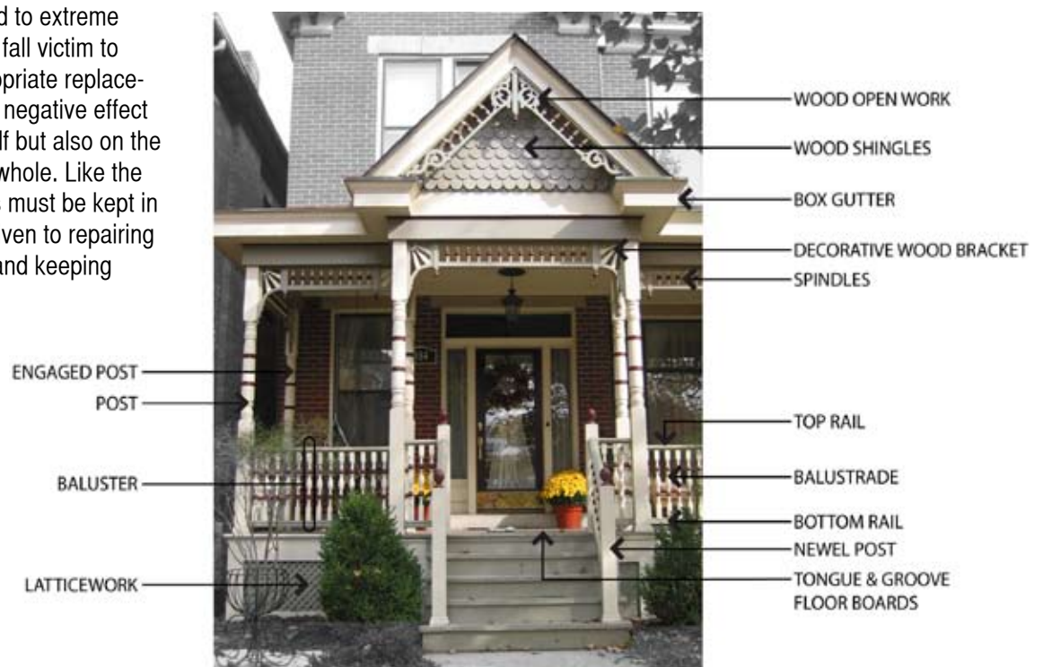
[ ILLUSTRATION 1 ] Parts of a Typical Porch
