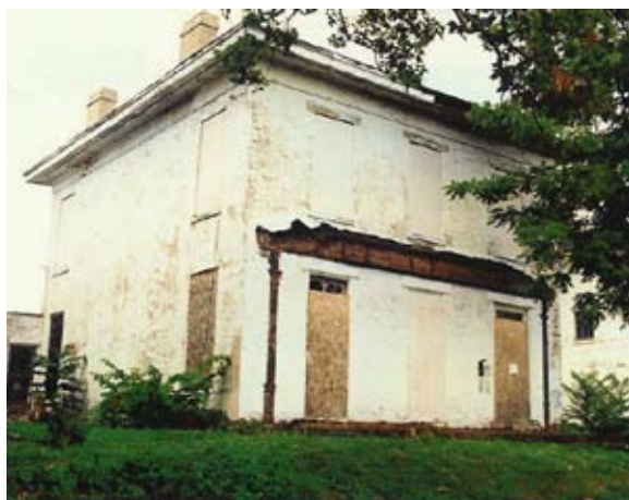
[ PHOTOS 8 AND 9 ] Before and after views show this S. Fountain Avenue house in 1995 and today. Paint shadows illustrate the profile of the original porch in the earlier photo. The new porch design makes use of typical porch characteristics for the period, including the chamfered posts and brackets, but keeps the elements simple.
