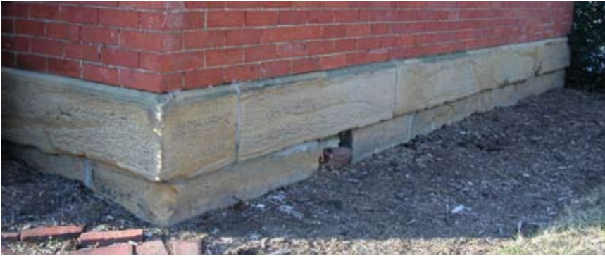
{PHOTO 1} A foundation of cut sandstone blocks that form a water table for this brick building.
