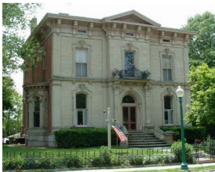
{ PHOTO 3 } Smooth finished stone used as facade treatment for this East High St. residence.
