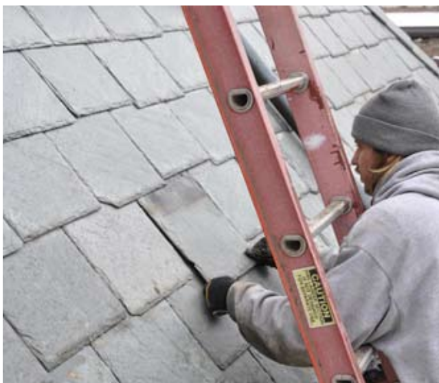
[ PHOTO 4 ] A workman replaces an individual damaged slate with a new slate that has been carefully selected to match the size, color and qualities of the original.
