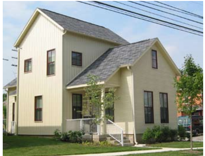
[ PHOTO 4 ] This example of new infill construction uses common proportions and roof forms in its historic area, but is clad in newer materials that recall historic materials. These include aluminum siding in two profiles (horizontal lap siding and vertical board & batten), aluminum-clad double hung windows, asphalt shingle roof, and split-face concrete block foundation.
