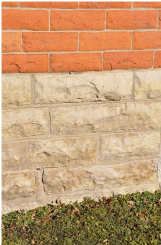
[ PHOTO 6 ] The masonry joints in this sandstone foundation have been carefully repointed to ensure the stability of the foundation wall.
