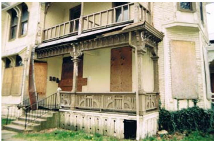
[ PHOTOS 6 AND 7 ] A porch on South Fountain Avenue before and after repair. The porch remains unchanged, with repair of damaged features and replacement of missing pieces to match the originals.
