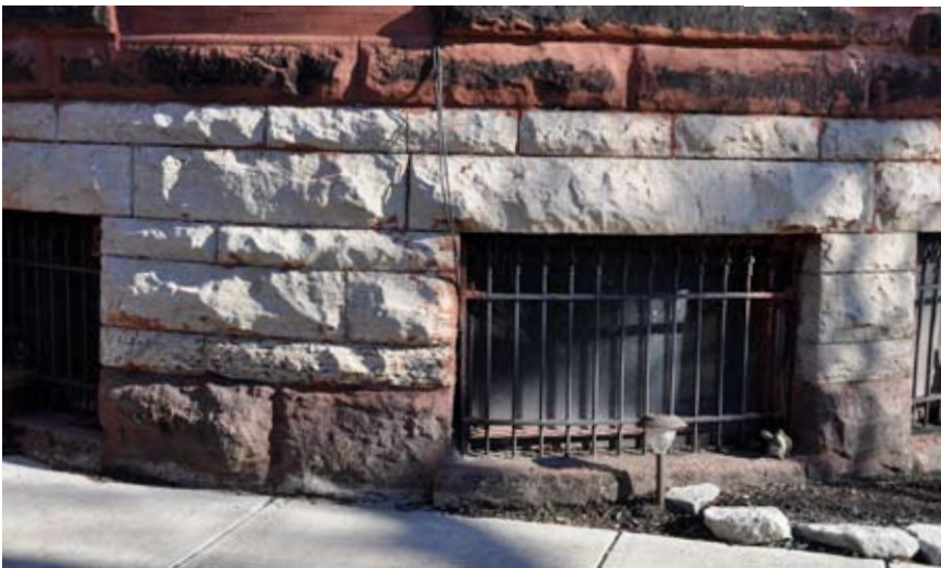
{PHOTO 2} Rock-faced sandstone blocks form a distinctive foundation on this 19th century home. Note the wrought iron security grille at the window opening.
