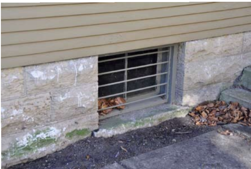
[ PHOTO 7 ] Simple horizontal or vertical metal bars would be appropriate security grilles for most foundation windows on historic buildings.
