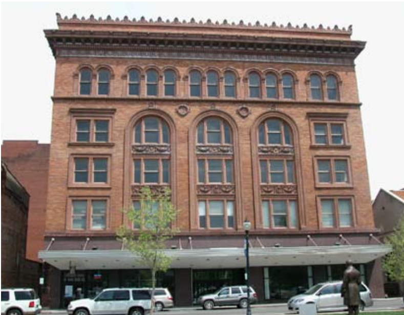
[ PHOTO 1 ] The Bushnell Building's upper facade is richly ornamented with arched windows, terra cotta trim, and an elaborate projecting cornice that crowns the building.
