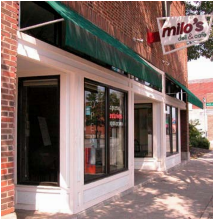
[ PHOTO 5 ] An example of a fabric awning mounted on an aluminum frame with open ends. This type of awning is a contemporary and compatible treatment for most historic commercial buildings.
