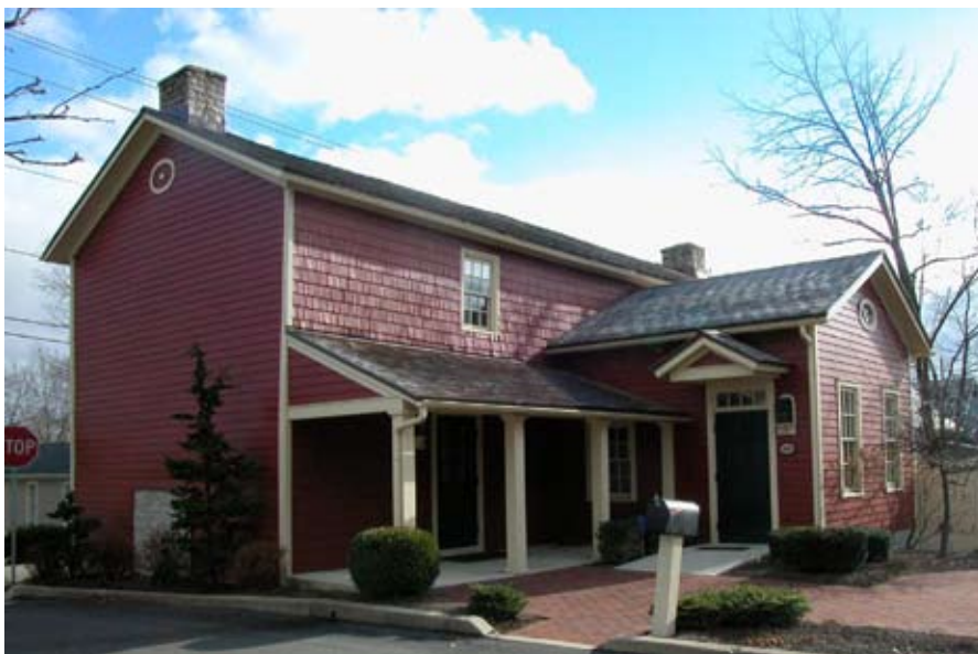
[ PHOTO 5 ] An example of an addition to the back of a property in a historic area. It is subsidiary to the original building, including its lower roofline, and is designed to be compatible with the simple style and materials of the original. The historic character and features of the original building remain intact with this addition.
