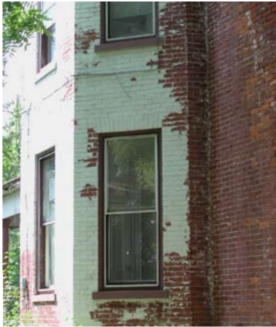
[ PHOTO 10 ] Paint removal from brick or stone can be difficult to achieve and is not always recommended. It must be carefully done to ensure that the masonry itself is not damaged.
