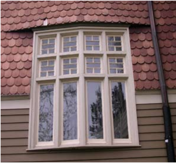
[ PHOTO 6 ] The transom (multi-pane) in this window is an example of a fixed window.
