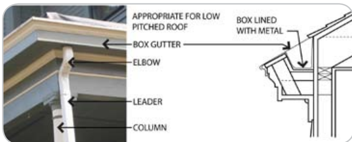
[ PHOTO 3 ] Box Gutter
