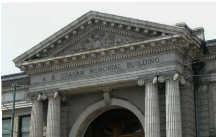
{ PHOTO 5 } The A. B. Graham Memorial Building exhibits elaborate terra cotta detail in its central pediment feature.
