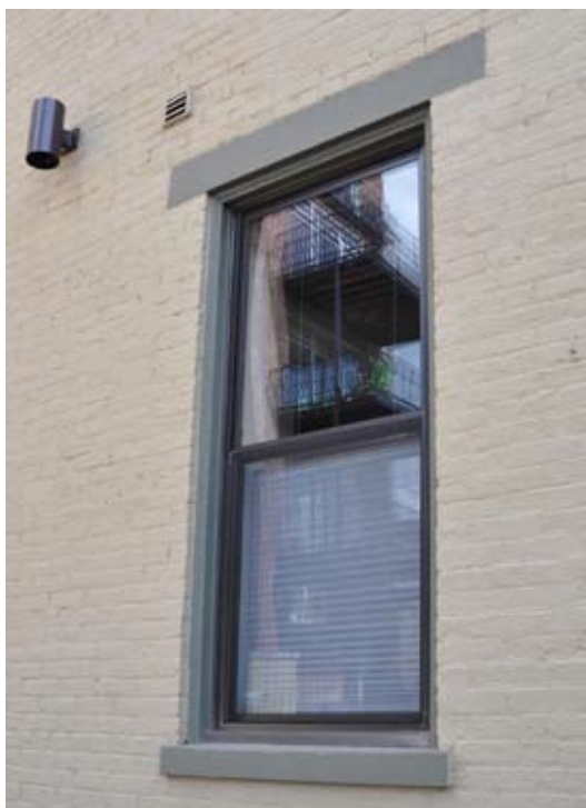
[ PHOTO 11 ] An example of an aluminum replacement window on a rear elevation of the building. Note how only the material is different; window still has the look of a wood window.
