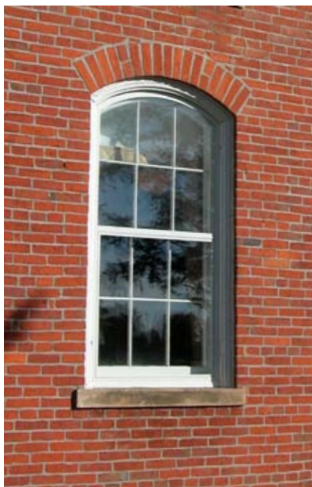
[ PHOTO 10 ] An example of a wood window replacement that matches the historic window exactly, including material.
