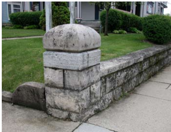
[ PHOTO 4 ] A limestone pier marks the corner of this property, with the retaining wall lining the property beyond.
