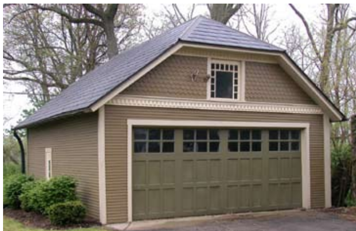
[ PHOTO 4 ] This frame 2-car garage has distinctive features, including a slate roof, wood shingles and wood shiplap siding. The double garage door has a traditional feel, with a combination of flat panels and small windows.
