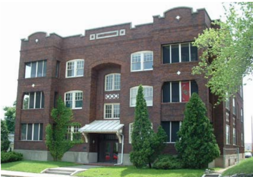
{ PHOTO 2 } This early 1900s apartment building is an example of brick used as a facing material, rather than as a structural bearing material.
