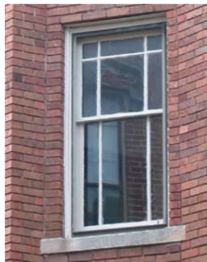
{ PHOTO 3 } An example of a double-hung window with patterned sash from the early 1900s.
