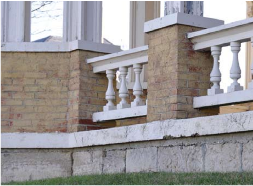
{ PHOTO 5 } — This porch foundation, with its distinctive stone water table, is an architecturally significant feature of the house and should be maintained along with the main building foundation.
