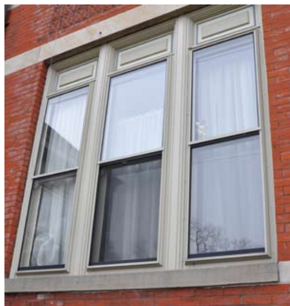
[ PHOTO 12 ] These storm windows fit the openings exactly, match the trim color, and provide insulating protection for the historic wood windows.
